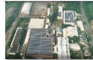
Solar Plant 1.3 MWp at M/s Timken
