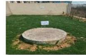
Rain Water Harvesting at M/s FFPL
